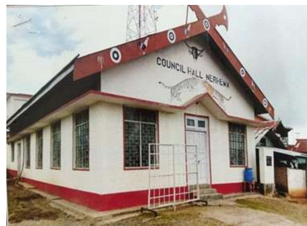
Construction of Council Hall at Nerhema village, Kohima
