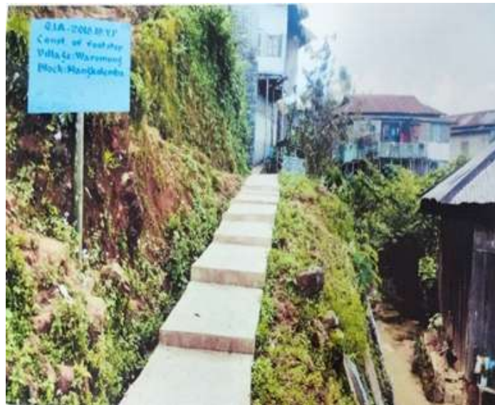
Construction of Footstep at Waremung Village, Mokochung
