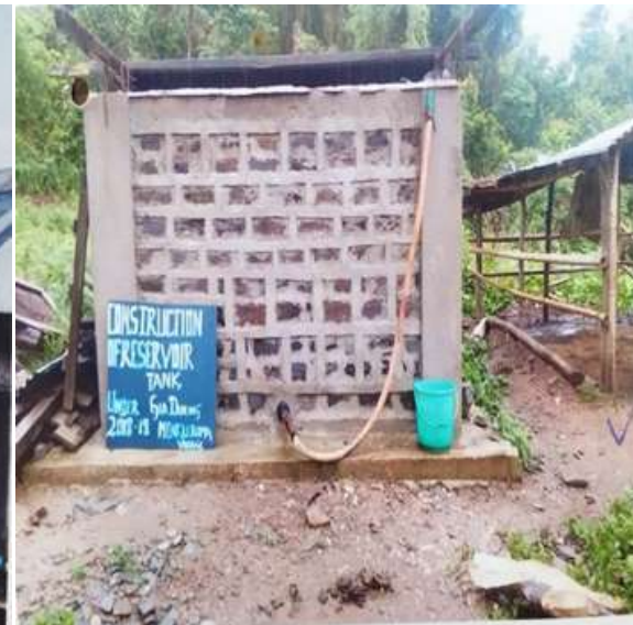
Construction of Water Reservoir at Mengujuma village, Kohima
