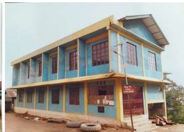
Construction of Multi-purpose Building Dzulhami village, Phek
